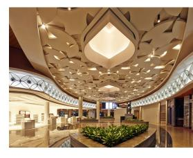
joints for building movement. Furthermore, due to the anticipated temperature differences between the Departure Hall and the plenum space above the ceiling, allowances were needed for ceiling expansion. With the pattern of coffers blending into the column capital, and 10 mm joints between all ceiling units, there was very little tolerance. These joints, in some locations, served as expansion joints.
